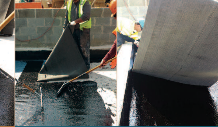
Layering BP Sheet into BP Primer•Adhesive
