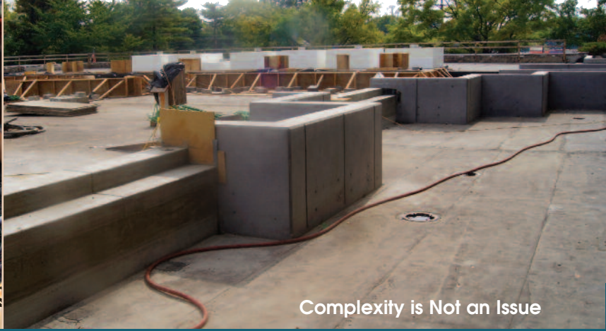
Mudslab and Foundation Walls
