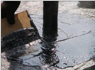
5. Apply hot bitumen around the base of the pipe, at least 12 inches out from the base of the pipe, completely embedding the star cut of the flashing sheet.
