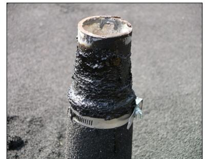
9. Install Ram 306 or 306M cap sheet in hot RT 250, seal the top edge of the sheet with RT 250 bitumen and secure with stainless steel clamp.<sup>1</sup>
