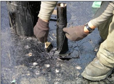
4. Seal lap with Ram-Tough 250 and press tightly onto place, making certain that the flashing sheet is tightly fitted at the intersection of the pipe and the deck.
