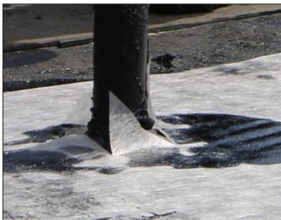
8. Install the primary horizontal Ram-Tough 250 waterproofing system over the flashing sheet and build-up slightly at the base of the pipe.
