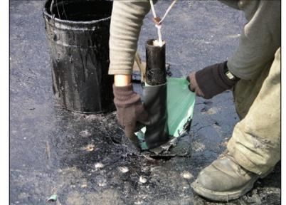
3. Before sealing lap with additional Ram-Tough 250, remove plastic separator sheet.
