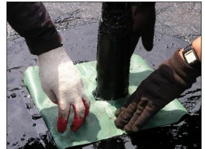
6. While the bitumen is still warm, slip a second ply of Ram Flash 327HDR, over the pipe, having it extend at least 6 inches out from the base of the pipe in each direction. Cut the center hole smaller than the pipe to obtain a snug fit.
