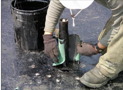
2. While bitumen is warm, wrap pipe with Ram Flash 327HDR 8 inches high, cutting base to flare out onto deck.
