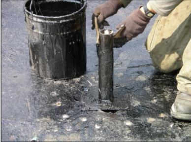
1. Before installing the waterproofing, clean metal pipe of all rust, process oil and other contaminants. Prime and allow to dry. Coat pipe a minimum of 8 inches high and the surrounding deck with Ram-Tough 250.
