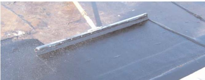
The preparatory work to all surfaces, cracks, joints, flashings, etc., must be completed as specified and the primed areas must be allowed to dry to a tack-free condition before the Ram-Tough 250 membrane is installed.
