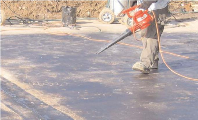
Apply Ram Primer/Surface Conditioner at a rate of 200-600 square feet per gallon, depending on the roughness and porosity of the concrete. Ram Primer/Surface Conditioner can be sprayed. If spraying, utilize spray equipment that can deliver the desired application rate without thinning the product. Mask all adjoining surfaces and avoid overspray. Avoid high wind applications unless adequate precautions are instituted.
