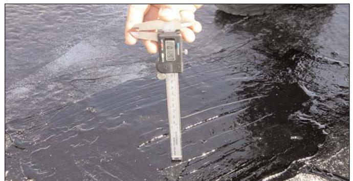
To determine if the proper thickness is being obtained, check the mil thickness with a common mil gauge and record the location and results.
