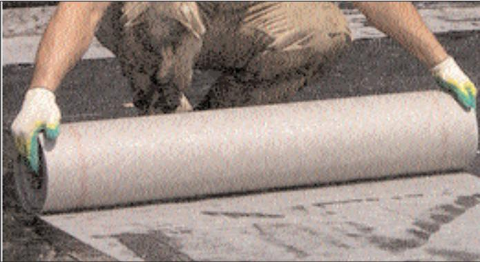
If it is necessary to walk over the completed membrane prior to the installation of the protection course, use Barrett Roof Release agent spray to create a bond break.
