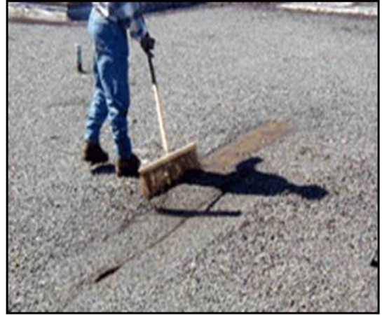
Step 8 – REPAIR SPLITS, RIDGES AND BLISTERS
