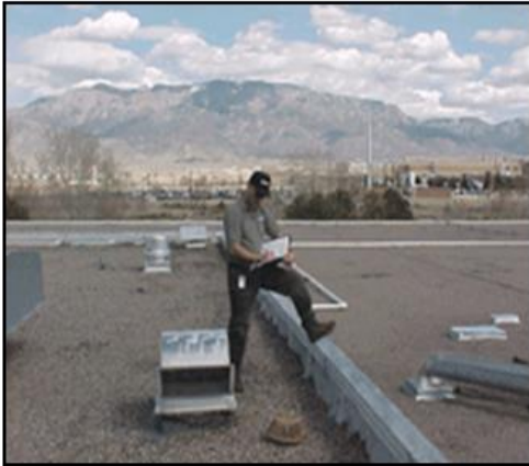
Step 1 – INSPECT ROOF
