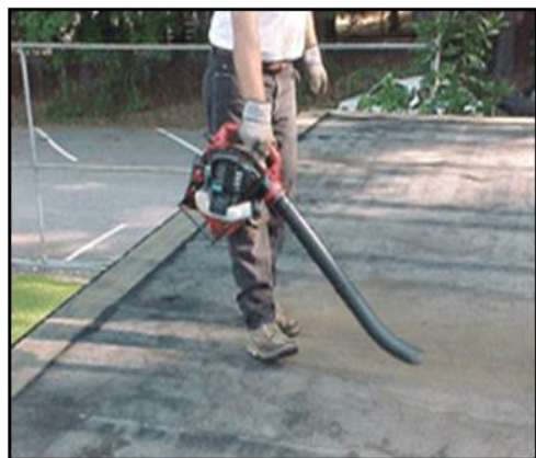
Step 6 – REMOVE REMAINING DIRT AND DUST
