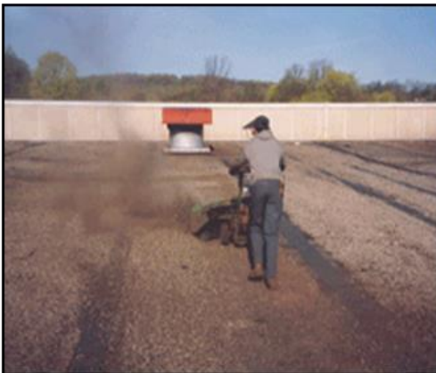
Step 5 – REMOVE LOOSE SURFACING MATERIALS
