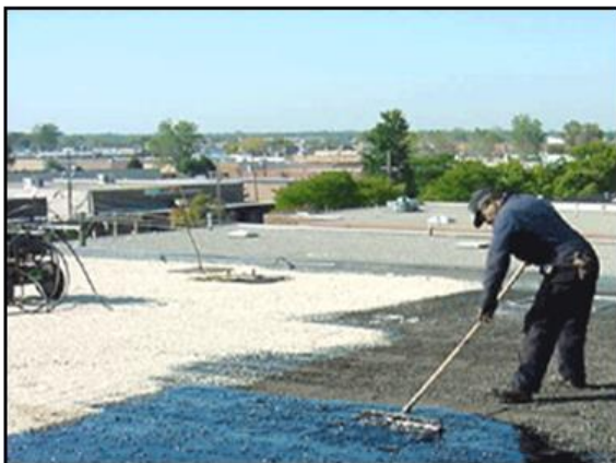
Step 16 – SPREAD WITH NOTCHED SQUEEGEE OVER GRAVEL, STRAIGHT SQUEEGEE OVER SMOOTH SURFACES
