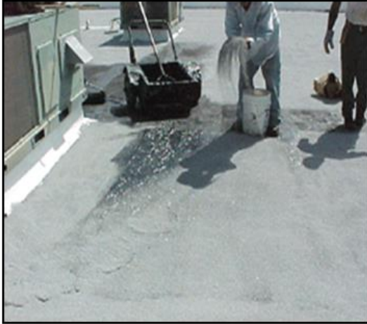
GRANULAR SURFACING
