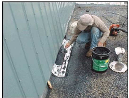
Step 12 – REPLACE OR RESTORE ALL BASE FLASHINGS AND PRIME ALL ASPHALT BASED ROOFS
