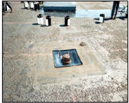
Step 10 – REFLASH ALL DRAINS
