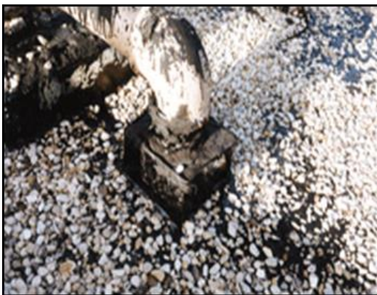
Step 11 – RESTORE MEMBRANE PENETRATIONS
