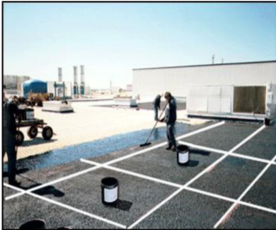
Step 13 – PLACE ram ColdTar ® PAILS IN GRID PATTERN
