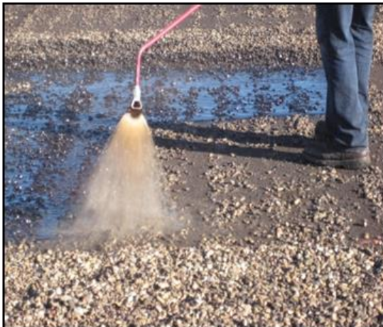
Step 15-A – SPRAY CLEANED MEMBRANE
