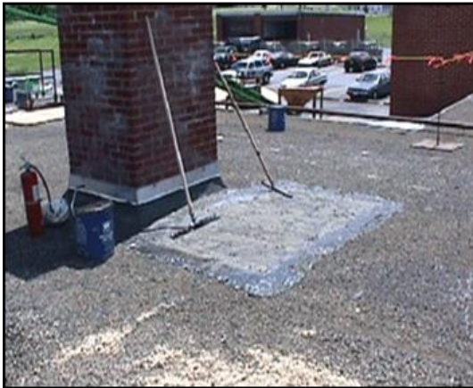
Step 9 – REPAIR ALL MEMBRANE DEFECTS
